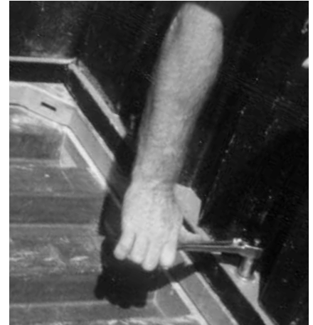
3 Vault assembles using only hand tools.
